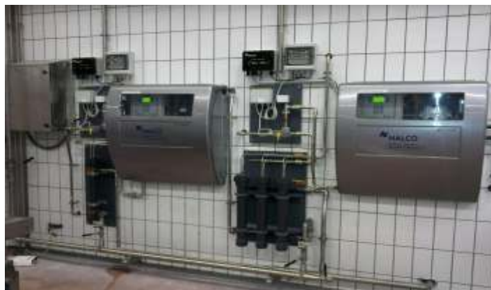
Nalco Water 3D TRASAR units in hot and cold legs of STORK hydrostatic sterilizer
