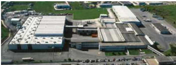
Figure 1: The Rieti Plant
