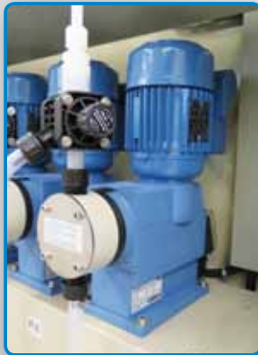
Ecolab diaphragm pumps with overpressure safety valves and/or snubbers against pressure shocks
