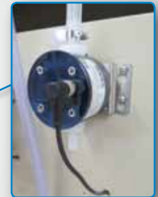
Dedicated flowmeter or oval gear meter for each product line
